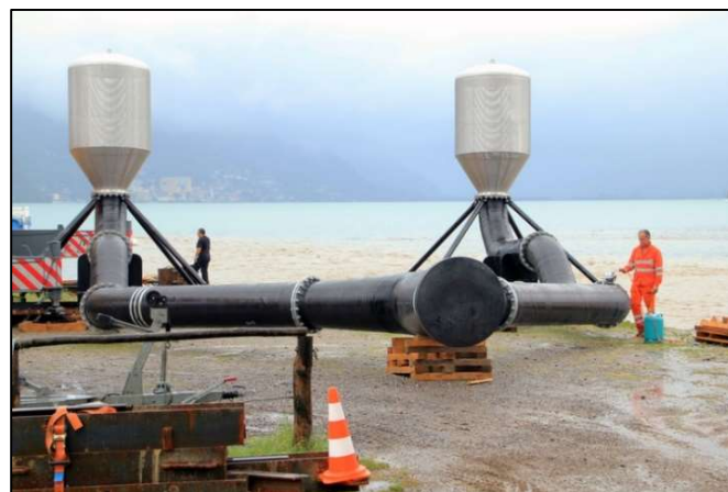
Figure 5-5 - Suction strainers for the lake water pipe before they were lowered 45 metres into Lake Lugano (picture: CSCS).
